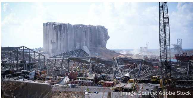
Photo 2: Destroyed buildings from Beirut's port explosion
